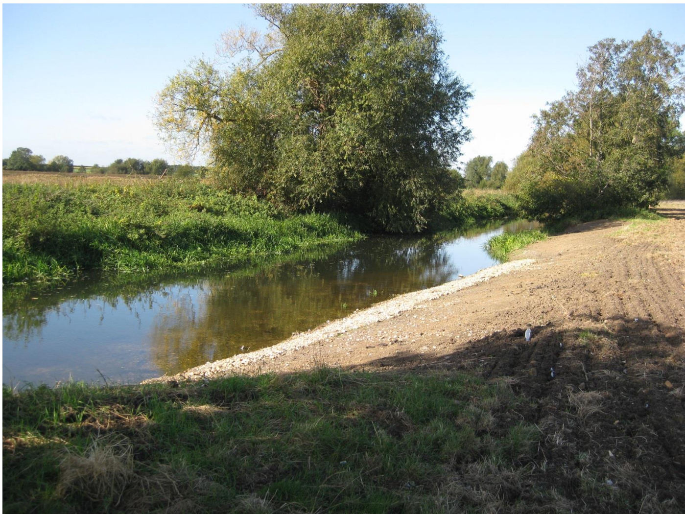
Figure 1 The new riffle at Trumpington Meadows
